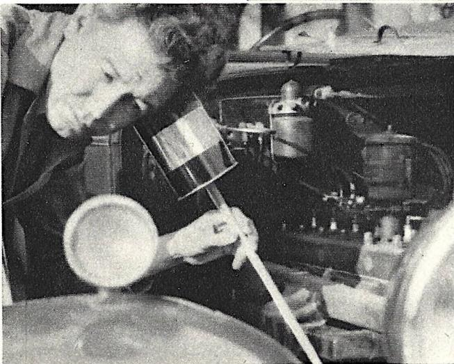
**H**ARD-TO-FIND noises can be located more easily by use of the motor stethoscope shown at the left. The device consists of a tin can open at one end, fastened by a nail through its bottom to a wood dowel about 18 inches long. Increasing loudness of the noise as the rod is moved near the defective part locates source of trouble.
