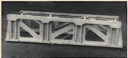
The unusual construction of the engine beds is illustrated in this plywood base. Note that plywood sides have been gauged out. Total weight is 40 pounds for each bed, reducing the weight over original beds several hundred lbs.
